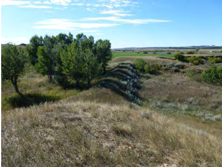
45. Dike at mouth of Fortune Coulee diverting flow to field to south.
